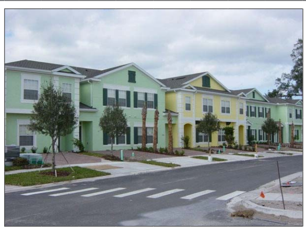
Block two at the Coral Cay Resort is nearly complete!
